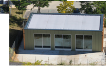
Façade test bench of Nobatek
