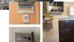
Demo building in Gdansk, Poland
