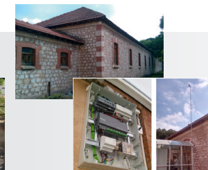
Demo building in Burgos, Spain
