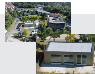
Façade test bench of Nobatek
