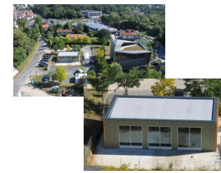
Façade test bench of Nobatek
