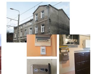
Demo building in Gdansk, Poland
