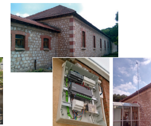
Demo building in Burgos, Spain
