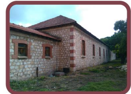
Demo building in Burgos, Spain
