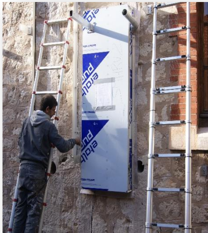
Installation of SMHRU
