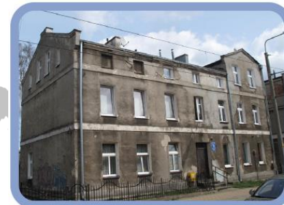
Demo building in Gdansk, Poland
