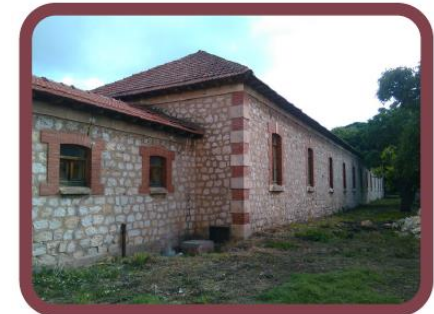
Demo building in Burgos, Spain
