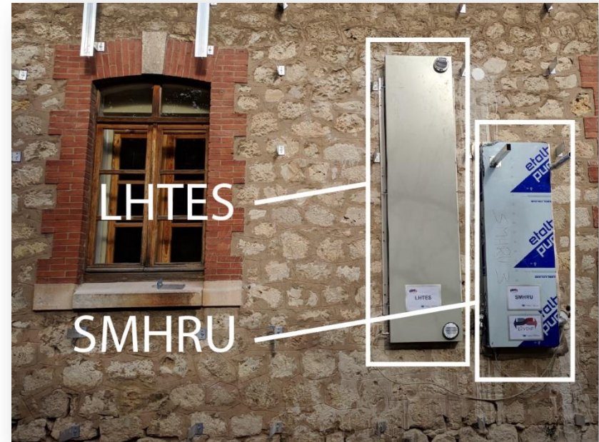
E2VENT system on the wall
