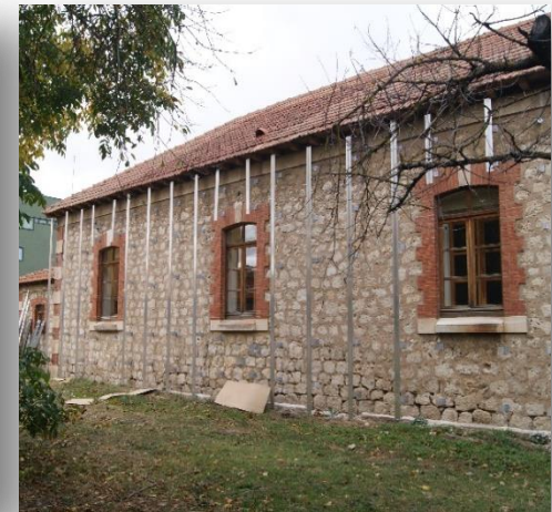
Anchoring + beams
